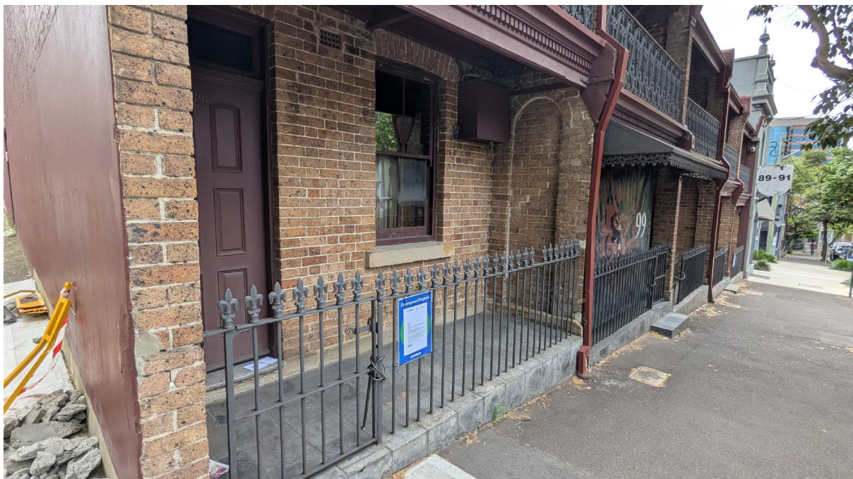
Figure 2: The front of the subject site viewed from Albion Street, looking west
