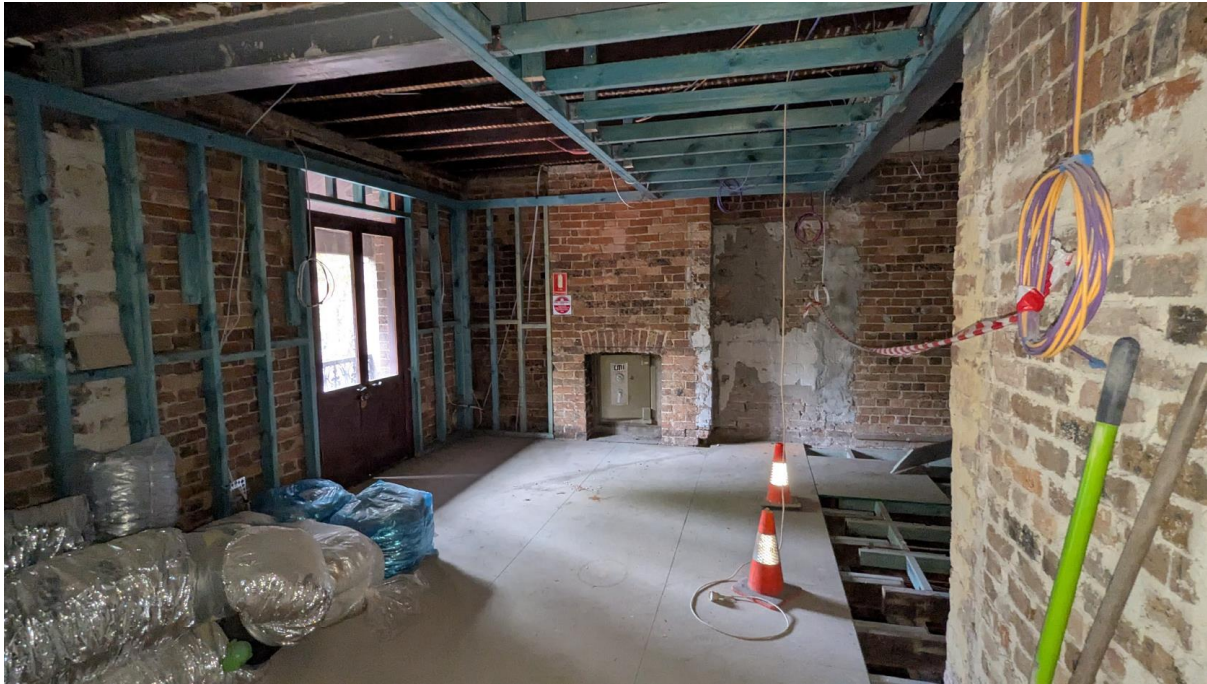
Figure 8: The current stripped and vacant condition of the interior of the premises, showing the retained original fireplace (being the first floor level of 95 Albion Street)
